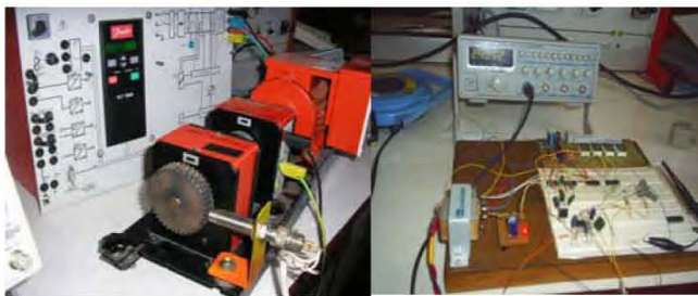
Fig. 11 Photo of Motor Drive with Speed Measuring Circuits
